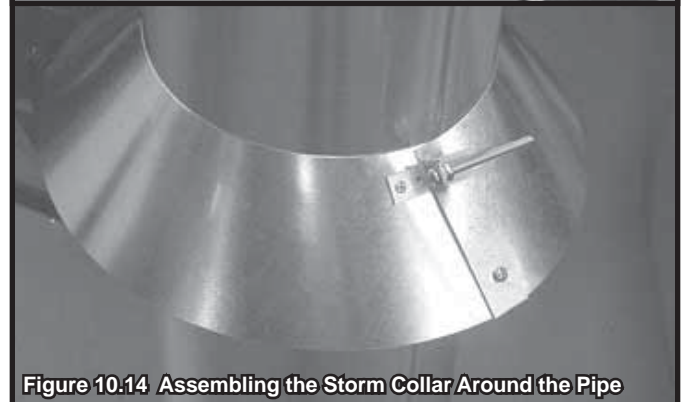
Figure 10.13 Assembling the Storm Collar
