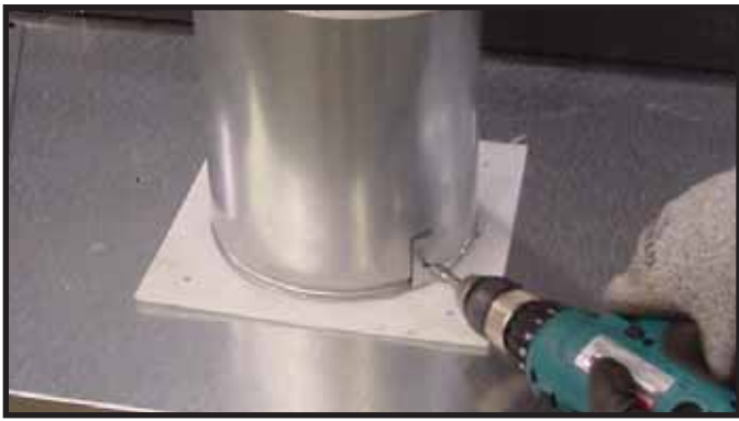
Figure 9.6 To attach the first section of vent pipe, make sure to use the fiberglass gasket in the manual bag to seal between the first vent component and the outer fireplace wrap. Use 2 tapping screws to secure the gasket to the outer wrap.
