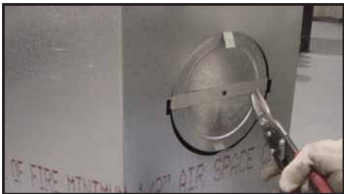
Figure 9.8 Cut the metal retaining band and fold the sides out.
