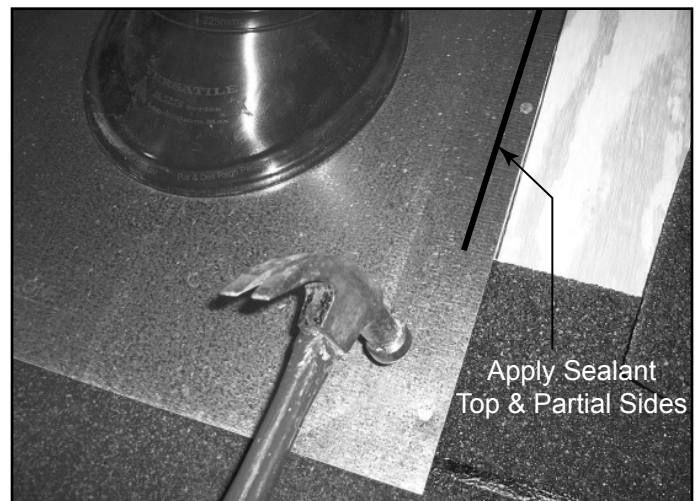
Figure 10.22 Slide Flashing Down, Secure & Apply Sealant
