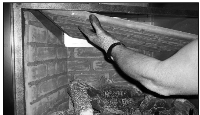
Figure 7.21 Remove Top Refractory
