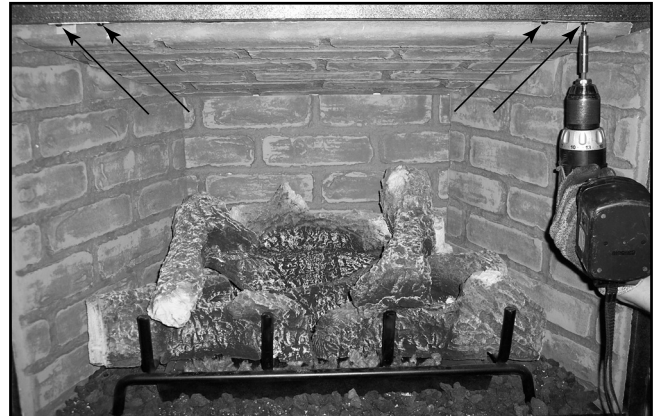
Figure 7.19 Remove Refractory Retainers
