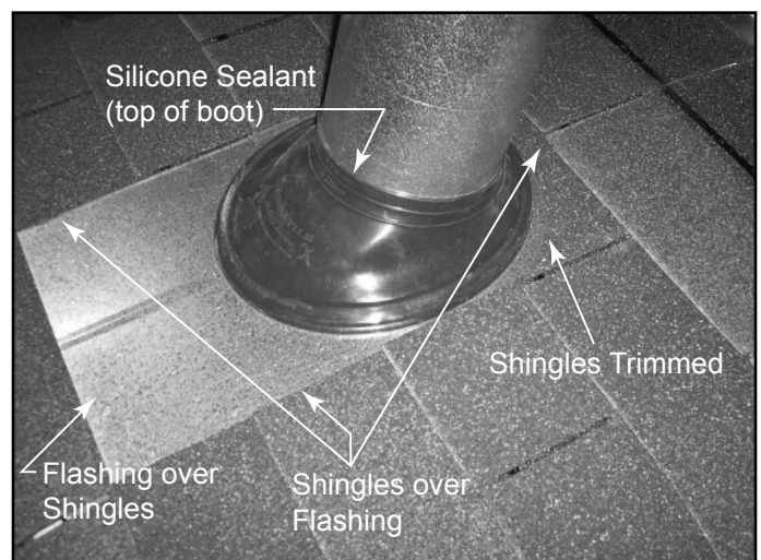
Figure 10.23 Installation Complete
