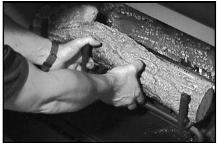
Figure 14.7 Remove Grate/Log Assy.
