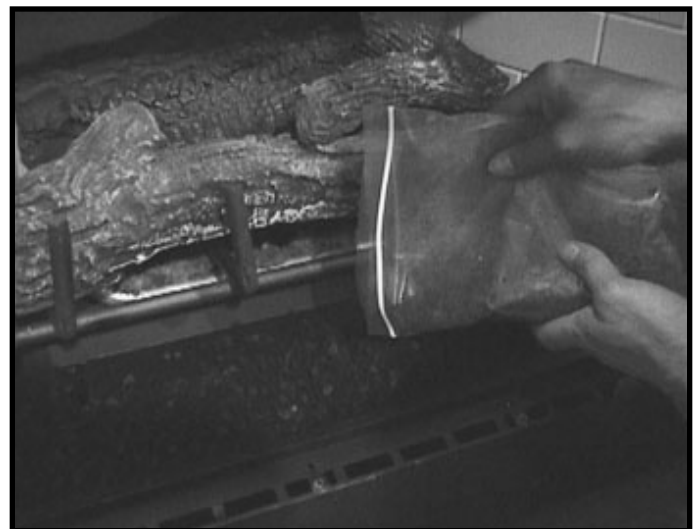
Figure 14.3 Placing the Lava Rock
