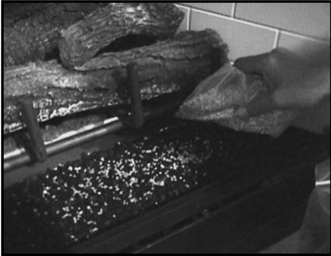
Figure 14.4 Placing the Vermiculite
