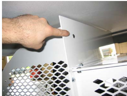
Attach ceiling filler panel to front partition using \frac{1}{4} " x \frac{3}{4} " carriage bolt and nut
