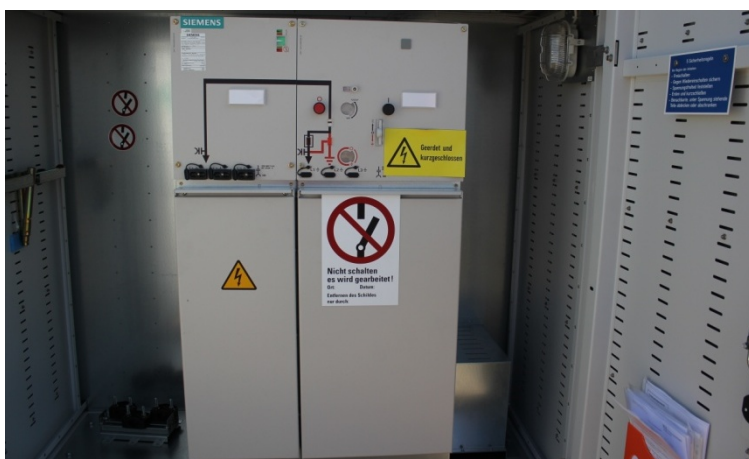
Figure 8 - MV switchgear (example)
