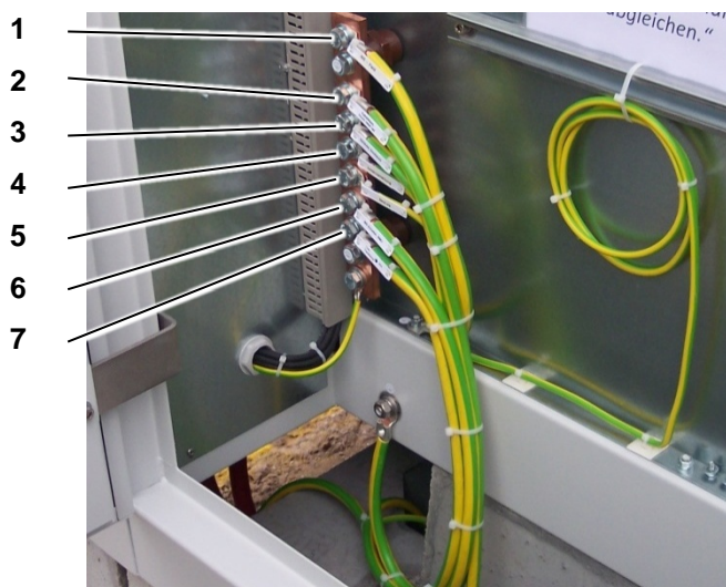
Figure 7 - Central earthing system (example)
