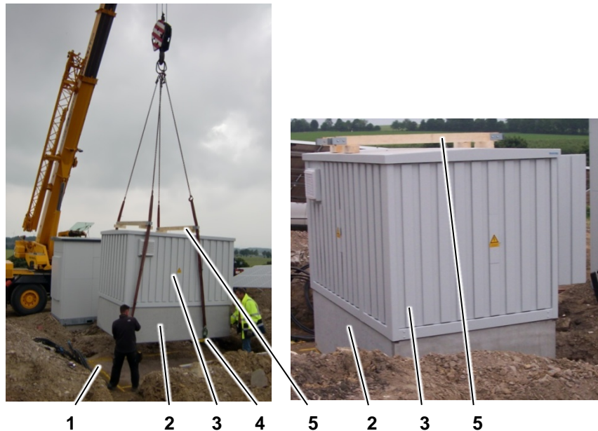
Figure 12 - Setting the compact station in place
