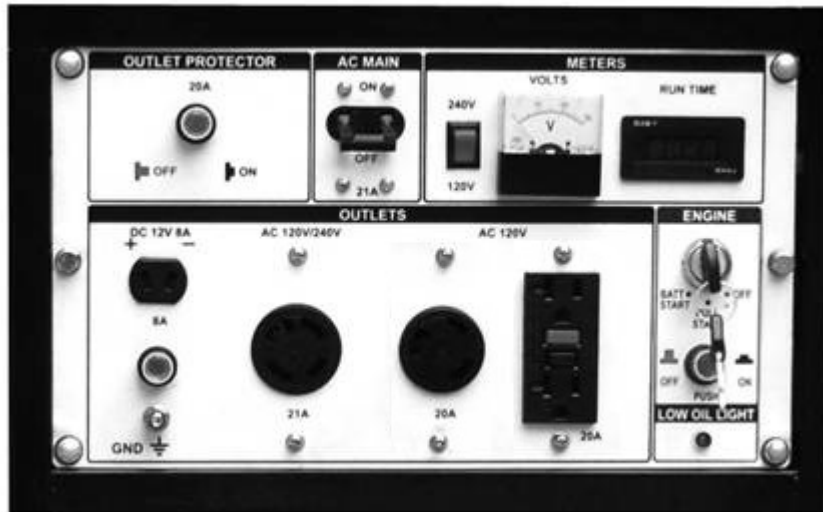
Figure 8 - Outlets Available on this Generator, from left to right, 12V DC, 240/120 AC (NEMA L14-30 plug) and 120V AC.
