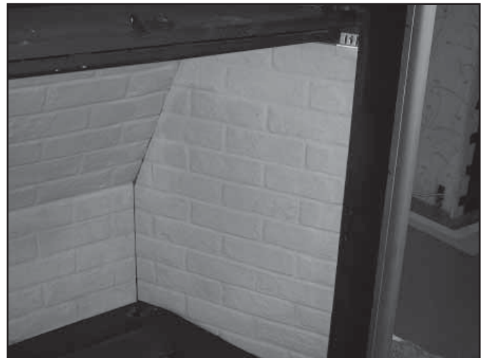
Figure 15.4 Install Right Side Refractory
