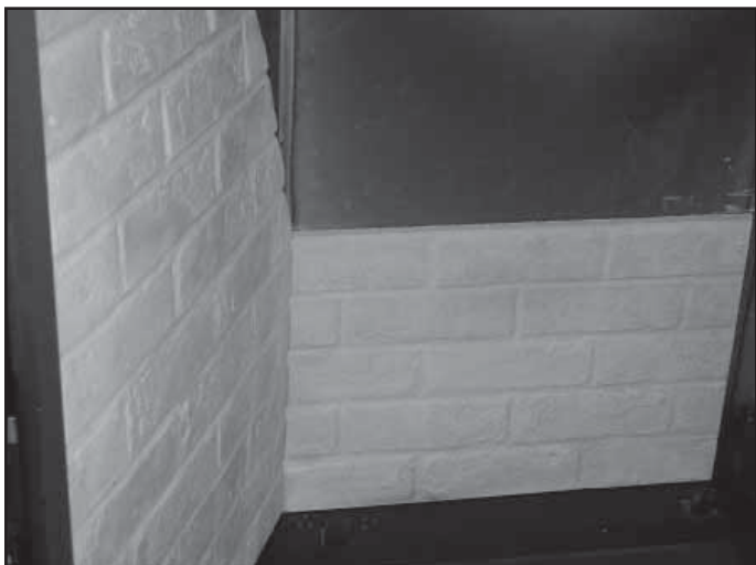
Figure 15.2 Install Lower Back Refractory
