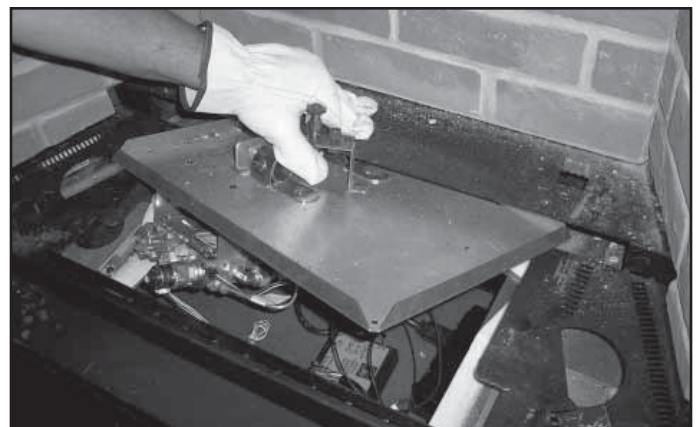
Figure 3.6 Lift Up & Remove Valve Assembly
