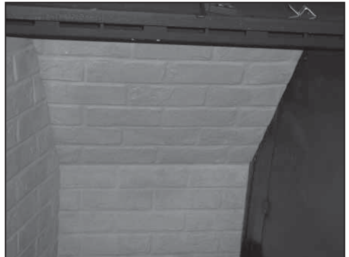
Figure 15.3 Install Upper Back Refractory
