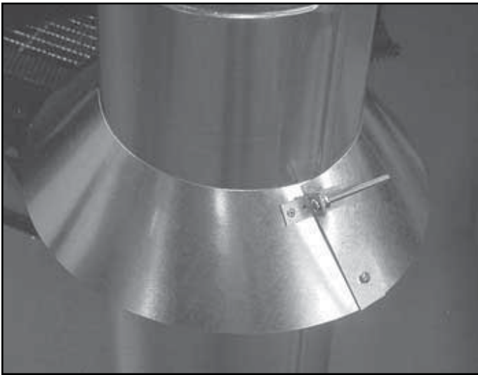
Figure 10.14 Assembling the Storm Collar Around the Pipe
