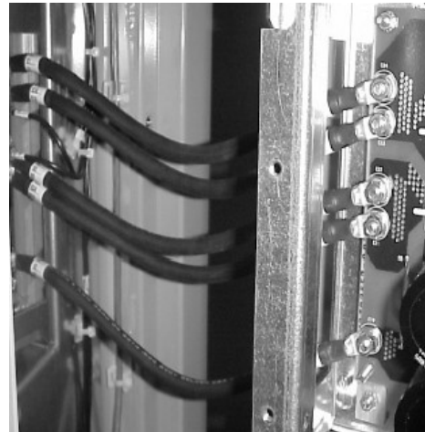
Figure 22: DC Bus Connections
