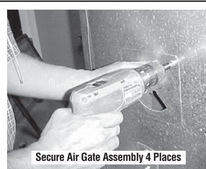
Figure 13 - Install Screws
