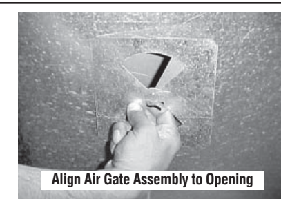
Figure 12 - Position Air Gate
