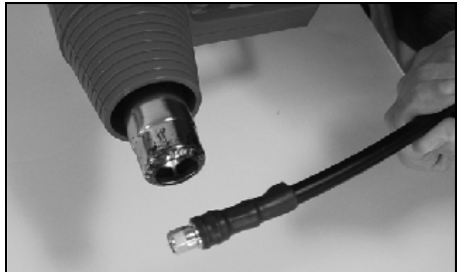
Figure 62: Applying the Heat Shrink Tubing
