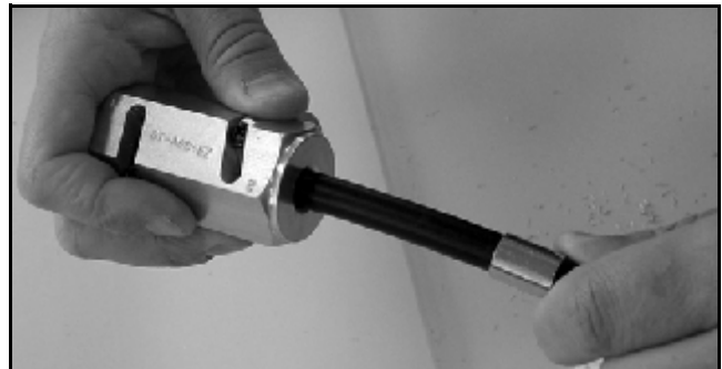
Figure 54: Stripping the Cable Jacket
